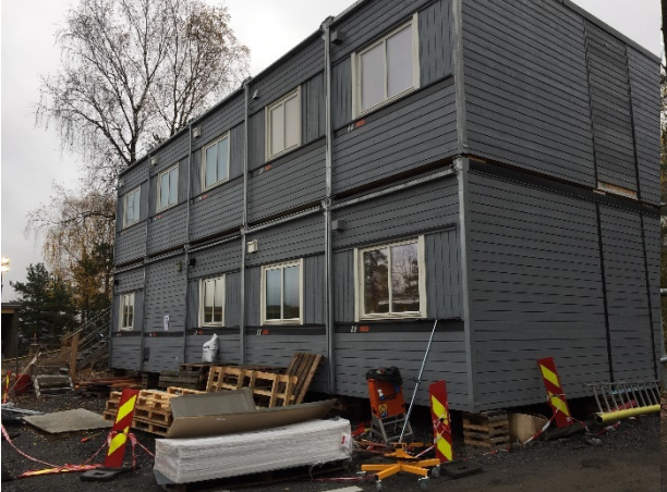
Modular offices, dinning and changing rooms
